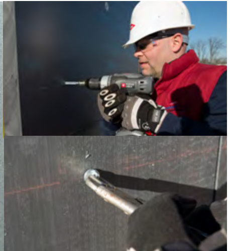
Note: If fastener is not in horizontal position, use a pair of pliers to rotate.
