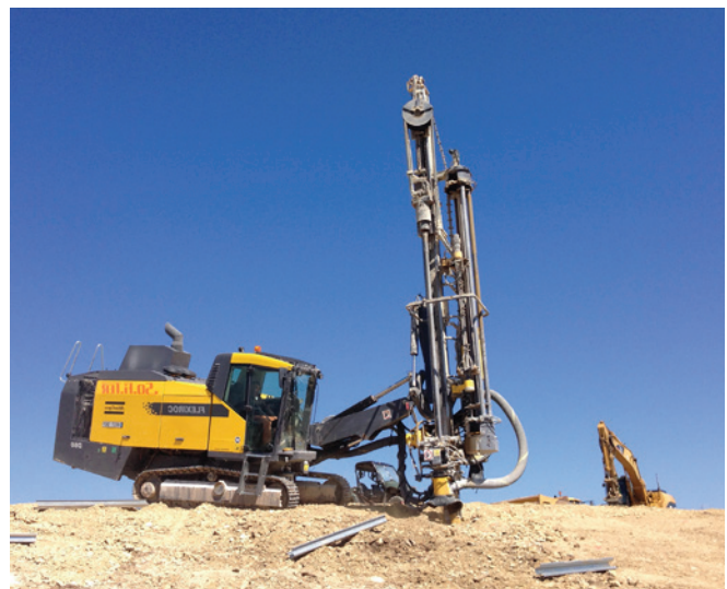
Rock breaker drilling holes for panel substructures
