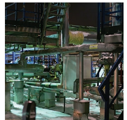
Hazardous maintenance operations
