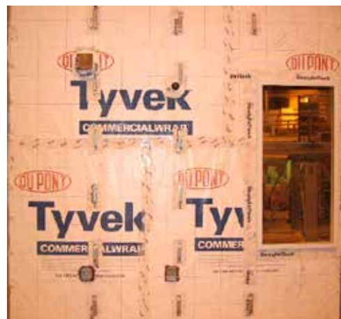
Figure 3: Penetrated Wall Configuration for ASTM E2357 Testing of DuPont™ Tyvek® Commercial Building Wrap Assemblies
