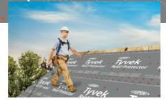
**Lightweight, Strong Roof Protection** Excellent grip to the deck and strength of product helps to minimize tearing at fastener points.
