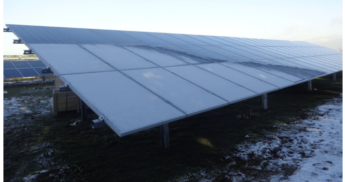
Solar panels coated in snow, during winter construction
