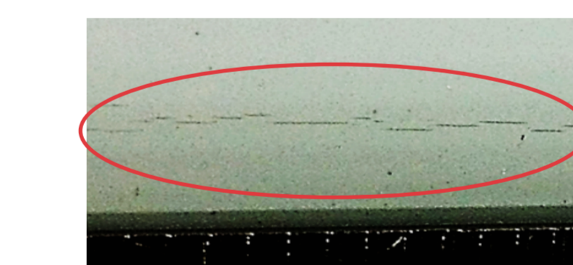
PVDF/PET/FEVE Backsheet Cracks of PVDF film found along ribbon after one thermal cycle.
