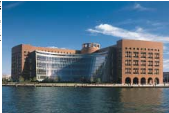
The Boston Courthouse's Conoid façade of laminated glass lets everyone inside – the judiciary and the public – enjoy the vista across the park and water to the city skyline.
