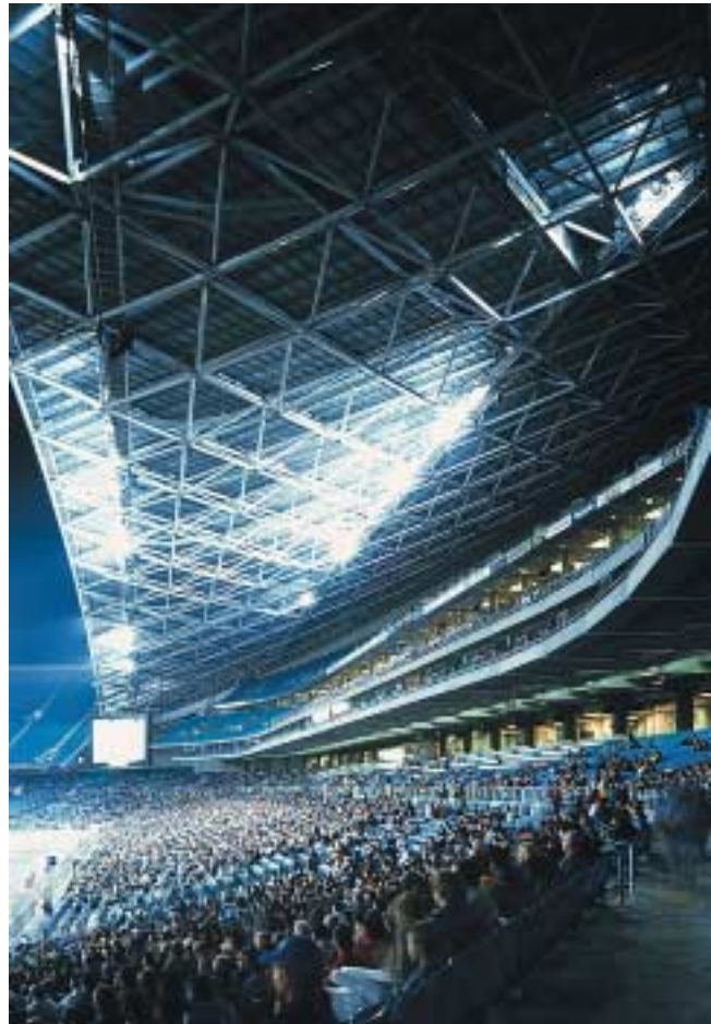
©Patrick Bingham Hall, courtesy of HOK + Lobb Laminated glass gives the press boxes in the world-class Stadium Australia optimum viewing and acoustic isolation.
