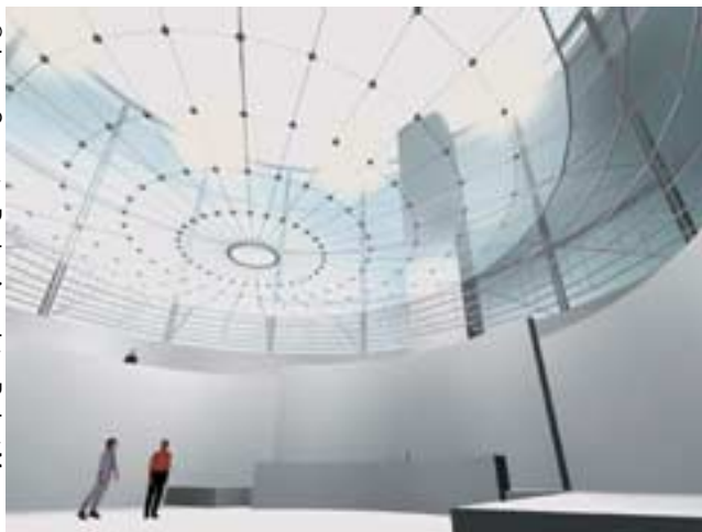
The award-winning lens ceiling of the Phoenix Courthouse incorporates DuPont™ SentryGlas® Plus ionoplast interlayer
