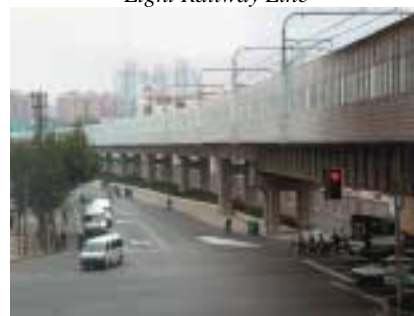
Shanghai Pearl Light Railway Line
