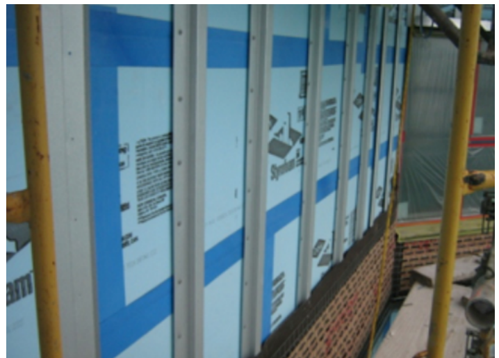
Photo 5b Galvalume Z-girts on 3" rigid XPS
