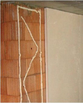
Apply adhesive to wall (or board)
