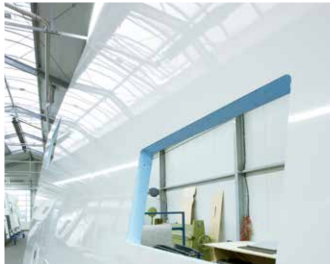
Fig. 15: The finished side wall
