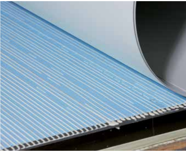
Fig. 12: Applying the glass fibre reinforced plastic outer layer
