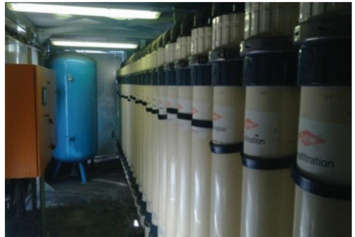
Initially, 60 Dow UF modules were installed, parallel to five sand filters to treat the water, which has since increased to three UF trains and 180 modules, completely replacing the sand filters. The UF-treated water is further processed by DOW FILMTEC™ BW30-400-FR Reverse Osmosis Elements to remove dissolved salts. Finally, the treated water is transported to a nearby power station, where it is demineralised with Dow Ion Exchange Resin Technology, and used as boiler feed make up water.
