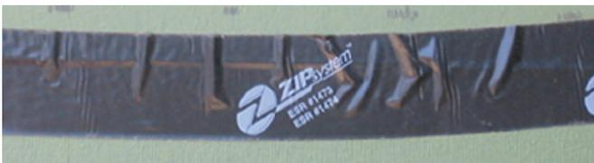
Proper taping is critical but can be difficult to achieve with the ZIP System®. Gaps, wrinkles, “fish mouths” and air bubbles create opportunities for water to enter the wall system. (Photo Source: Parksite)
