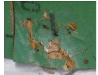
Over-driven nails cause damage to the WRB overlay of the ZIP System®, creating opportunities for air and moisture to enter the wall system. (Photo Source: Parksite)
