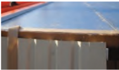
DuPont™ Thermax™ Insulation with Weathermate™ Flashing Applied
