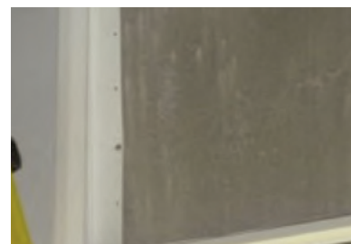
PVC attached to tilt-up wall
