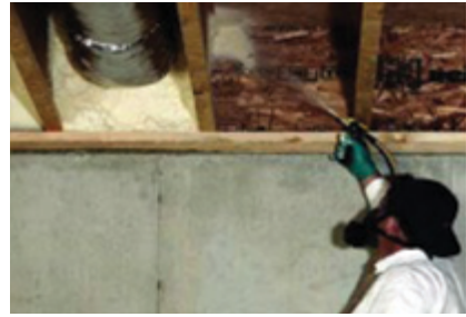
Applying an initial bead of foam where the rim joist meets the subfloor is called "picture framing."
