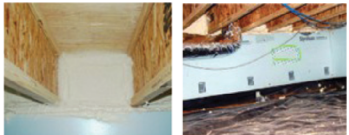
Typical applications of Froth-Pak™ Foam Insulation in rim joist areas.
