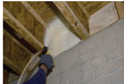
After picture framing, spray rim joist area to a maximum of 2" thick.
