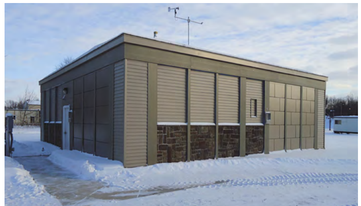
Wall Assembly Research Center: A laboratory built by The Dow Chemical Company in Midland, Michigan to test the performance of several different wall assemblies in real world conditions.
