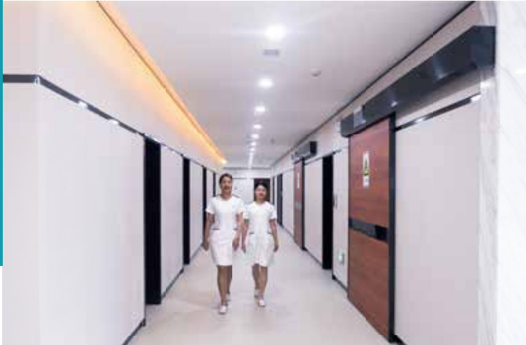
▲ Metal panel laminated with Tedlar® wallcovering in corridor
