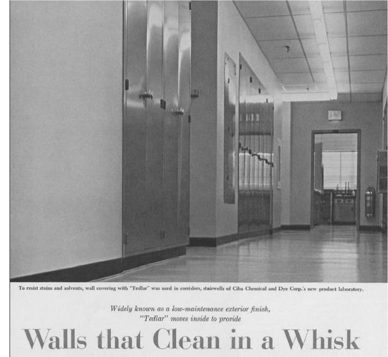
To resist stains and solvents, wall covering with "Tedlar" was used in corridors, stairwells of Ciba Chemical and Dye Corp.'s new product laboratory.
