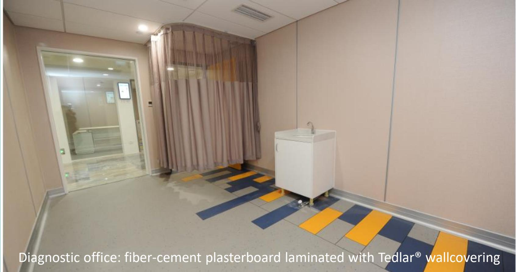
Diagnostic office: fiber-cement plasterboard laminated with Tedlar® wallcovering
