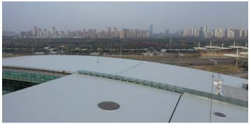
At the time of completion in 2004, the Shanghai International Circuit was the most expensive circuit facility in the world, costing \$240 million USD. The roof was originally PVDF coated aluminum, which had begun to crack and peel away from the roof in recent years.
