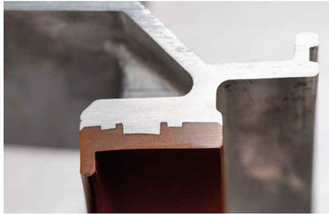
FIGURE 6 Cross section of bearing seat with Vespel insert (© DuPont)
