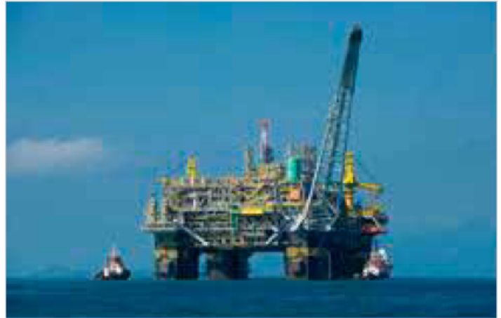
Offshore oil platform
