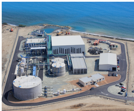
Air view photograph of Limassol Desalination plant. Courtesy of MN Limassol Water Co
