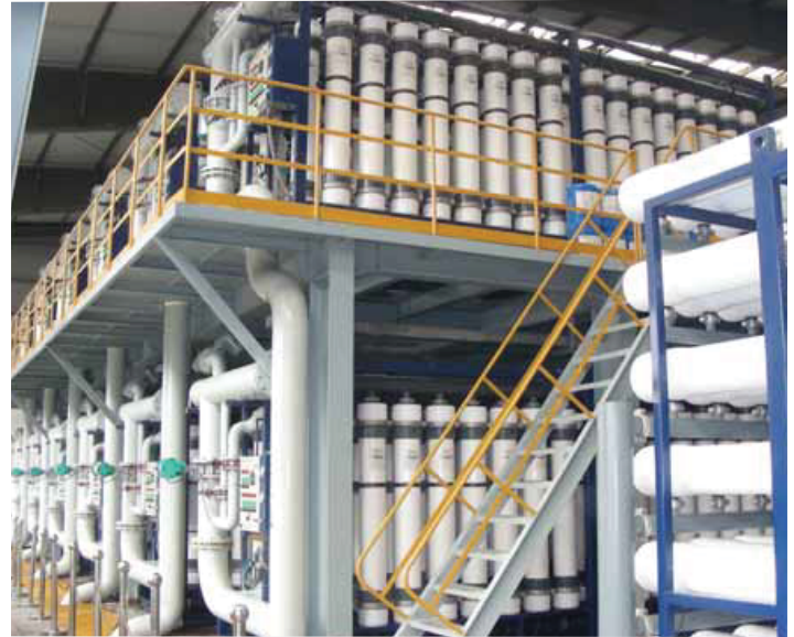
Two-floor arrangement of DuPont™ Ultrafiltration SFP-2860 modules in the Taiyuan facility. (Photo courtesy of Taiyuan Steel Group Co. Ltd.)
