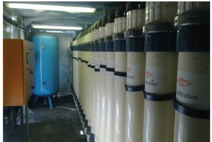
As conventional sand filters and other ultrafiltration (UF) technologies initially used to treat the mining wastewater were found to be ineffective, the coal mine turned to Dow Water & Process Solutions for UF technology as a pre-treatment to Reverse Osmosis (RO), to effectively recover wastewater.
