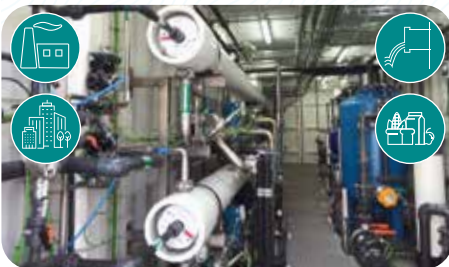
Closed Circuit Reverse Osmosis plant (CCRO-8)
