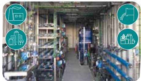
Closed Circuit Reverse Osmosis plant (CCRO-2.5)
