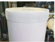
c) Put the 4<sup>th</sup> module on the interconnector of the 3<sup>rd</sup> module and push the package carefully into the pressure vessel (30-50 cm should remain outside)
