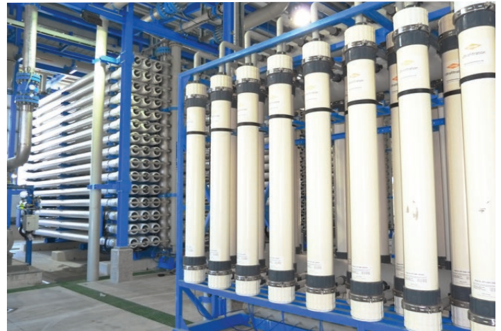
Photograph of a UF and RO train from Limassol Desalination plant. Courtesy of MN Limassol Water Co
