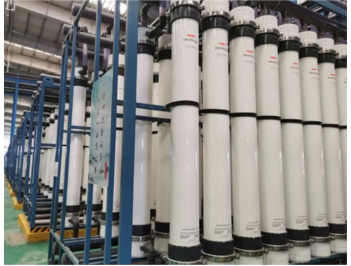
FilmTec™ Fortilife™ RO/NF product series are widely used in the whole process of this project, including CR100, XC70, XC80, ultra-high pressure reverse osmosis elements and XC-N nanofiltration elements. The state-of-the-art anti-fouling technologies implemented by FilmTec™ Fortilife™ elements ensures the efficiency and stability of RO system operation for treating the most challenging coal chemical wastewater.
